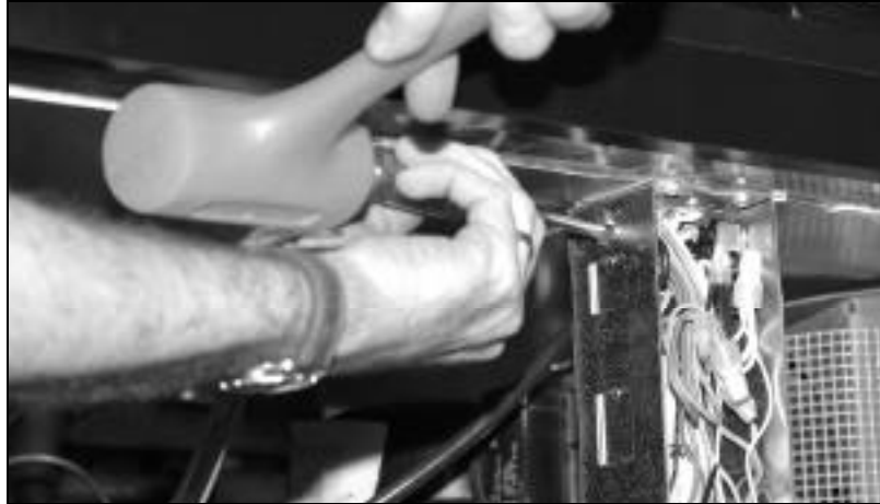
Figure 3. Driving out knockout
