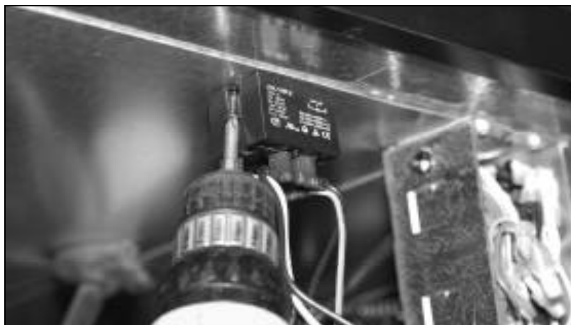
Figure 5. Anchoring relay
