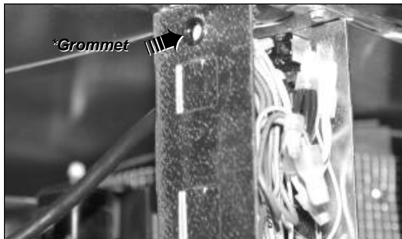
Figure 4. Installing the grommet
